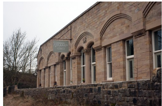
Hassop Station Tea Rooms
